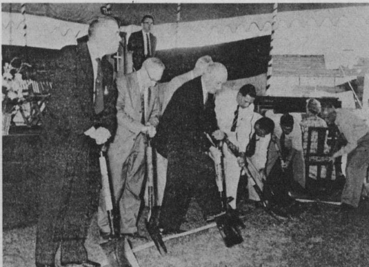
Ground-breaking service for the English-language church in Calcutta. The C.A.'s in America raised $20,000 for this building.
