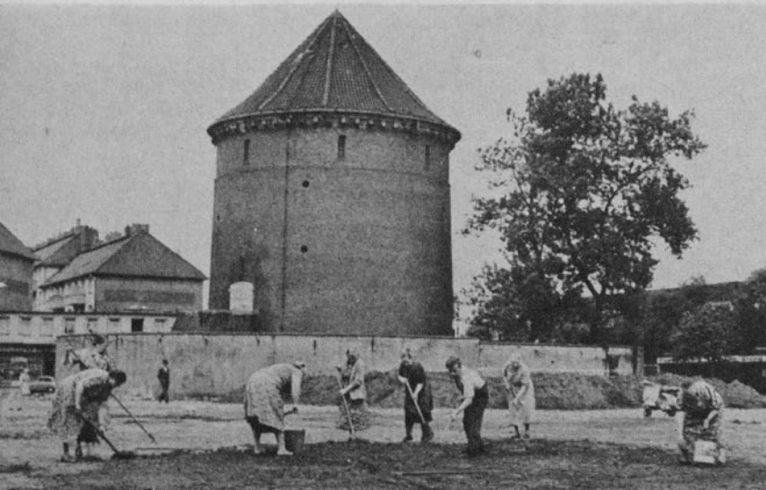
Preparing ground for tent at Hamburg. Tower is an air-raid shelter.
