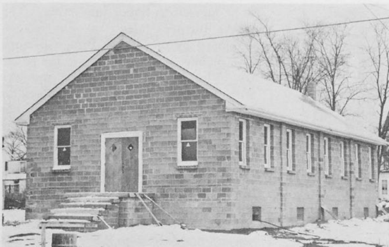
Hightstown Assembly under construction; P. Gibilisco, Pastor
