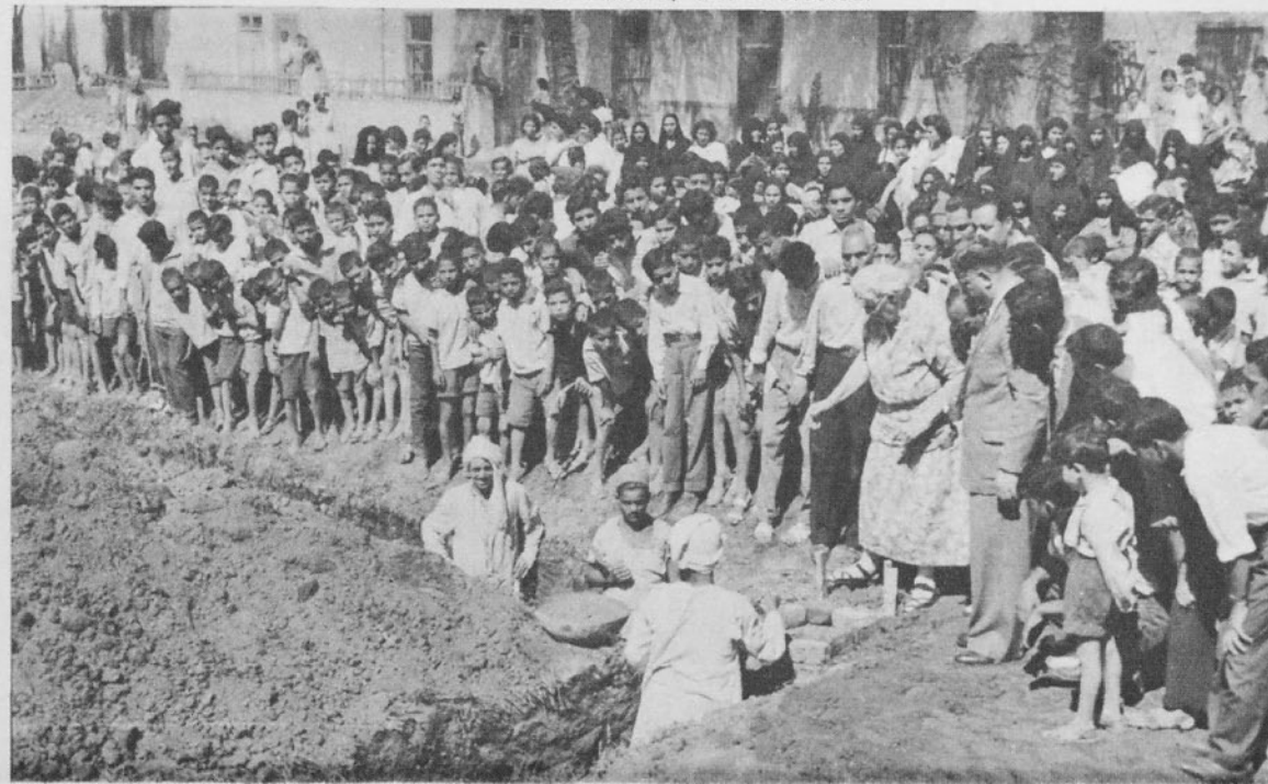
Laying the cornerstone of the new building. The foundation has been laid and as funds are sent in the building will be erected.
