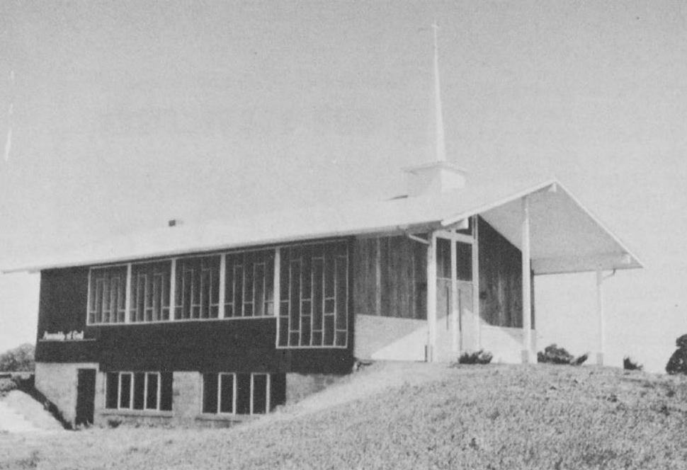
New church at Whitewater, Wisconsin, built from "The Herald" plans.
