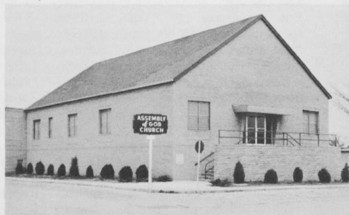
Church at Cushing, Oklahoma, after remodeling.
