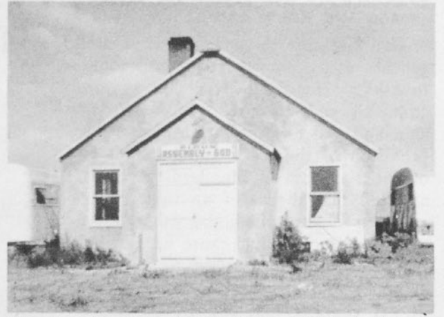
The Sioux Assembly of God, Norris, S. Dak., built from two donated barns with volunteer labor.
