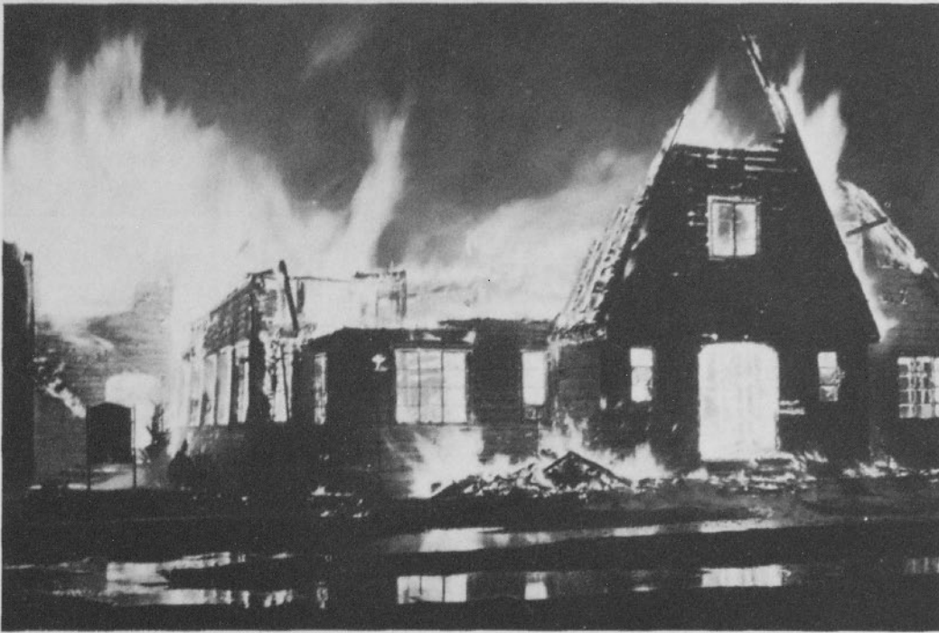
The Broken Arrow Assembly of God was destroyed by fire.
