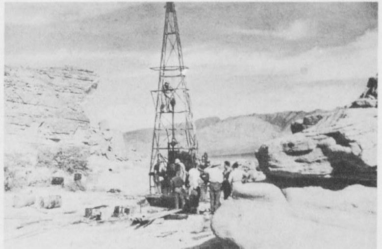
Setting up machinery to exploit the copper resources of King Solomon's Mines
