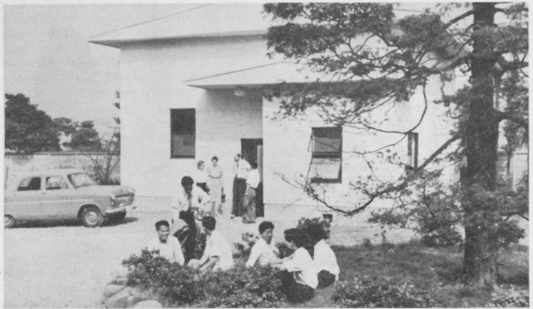
A view of the new Radio Studio from the Administration Building
