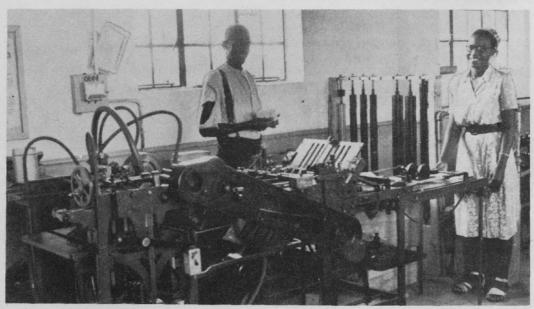
"Speed-the-Light" funds contributed by the C.A.'s in America furnished this automatic folding machine for Emmanuel Press. It operates at the rate of 9,000 folds per hour.
