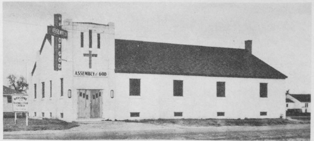
NEW CHURCH DEDICATED AT ROCK FALLS, ILLINOIS
