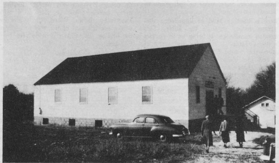
The new Assembly of God at Cave Springs, Mo.
