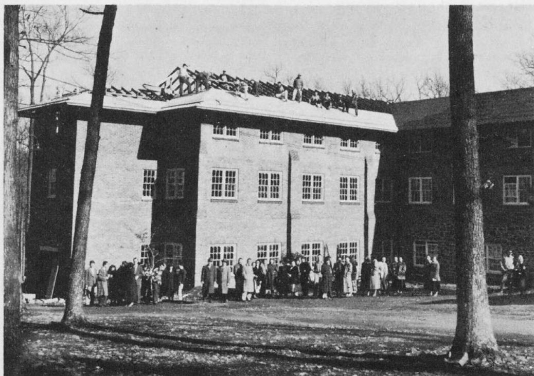
New Wing at Eastern Bible Institute Under Construction
