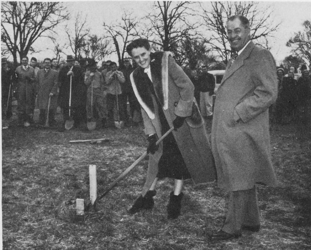
Sister Pauline Mastries, pastor of Bethel Assembly (formerly Northeast) of Springfield, Mo., turns the first shovel of dirt in ground breaking ceremonies held April 5, 1952, while K. H. Lawson, District Superintendent, looks on.
