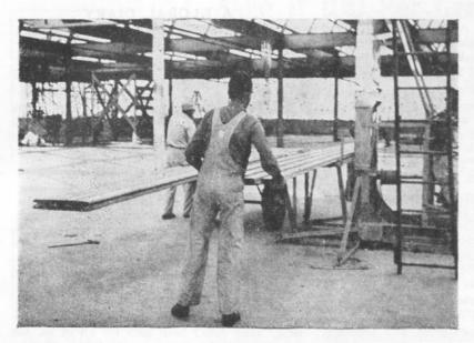
Workmen lay the heavy cue panels on the elevating platform of the Highlift machine, in preparation for their hoisting to the roof.
