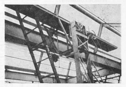
With the platform at the proper level, a rope is pulled to roll the cue panels off the Highlift machine and on to the roof. They are quickly spot welded in place, and will form the base of the roof material.
