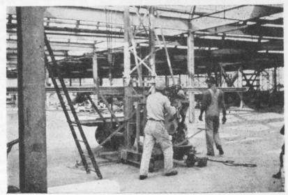
The cue panels are heavy, but turning the crank lifts them rapidly to the roof level. Workmen take turns cranking the machine.
