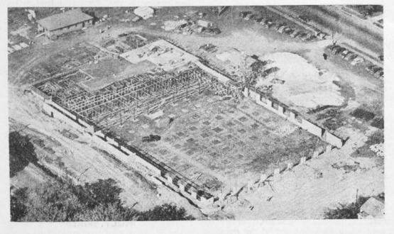
poured concrete. It is being worked on; perhaps you can see the concrete smoothing machine being run by two men. Other men are on their knees with their trowels, finishing off the wet concrete.
