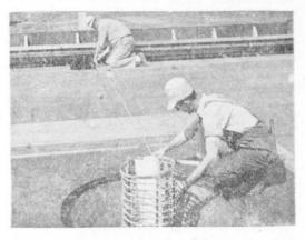
With the figures in mind as the blueprint calls for them, careful measurements must be made. Everything must measure out to the fraction of an inch. The workman in the foreground is in the section over the top of a pillar. Notice the circular reinforcing steel bars protruding from the pillar.
