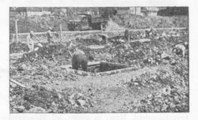
Workmen dug the footings with pick and shovel in preparation for the concrete foundations which will carry the weight of the great presses.
