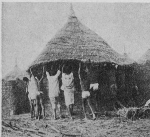
Raising the roof
