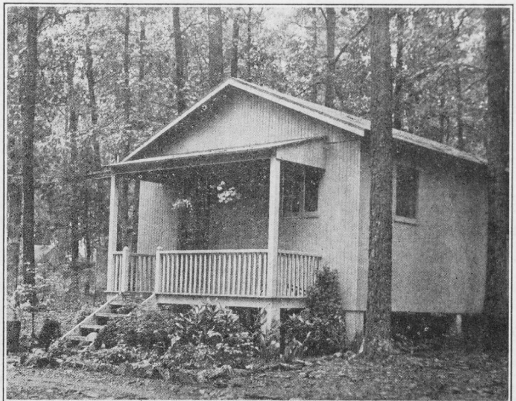
Typical Cottage, Green Lane Camp, Eastern District
