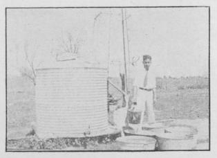
Catching water brought up by windmill power. Elevated tanks would eliminate this work and a student's time.
