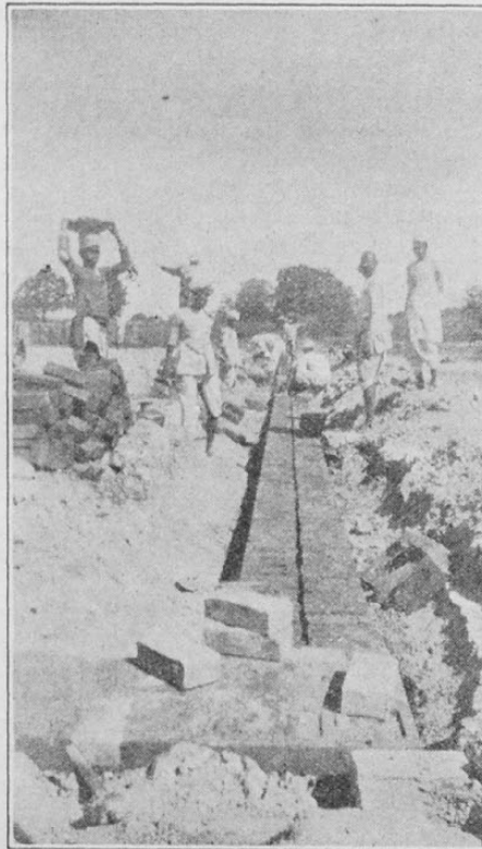
Laying the foundation of the walls for the women's quarters, of the Assemblies of God Bible School in North India.
