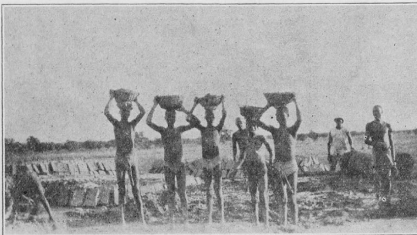
Building a house in Yako, French Sudan. The men are carrying mud in their baskets for mortar and brick making
