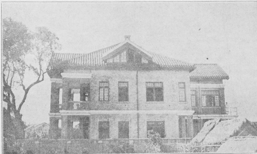
THE NEW RECEIVING HOME AT SAINAM, S. CHINA Recently Erected by Bro. Geo. Kelley. A Further $1,000 Still Required. Let's Finish the Job.
