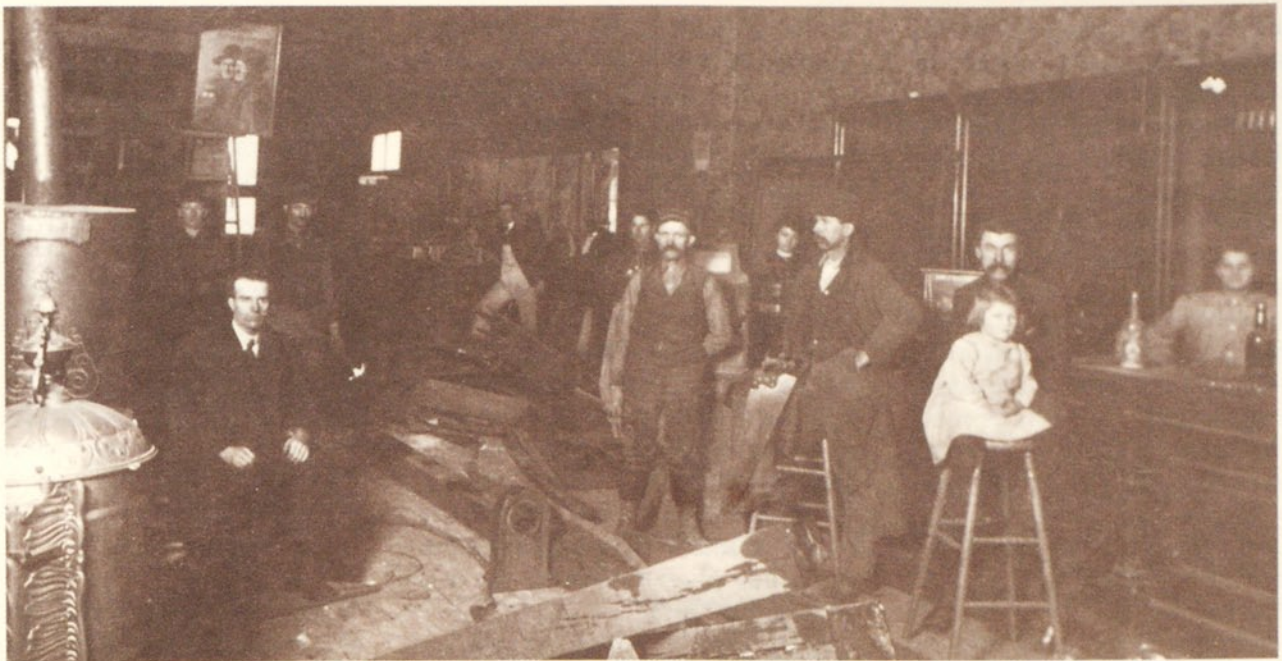
Here an old Findlay, Ohio, saloon is in the process of renovation for a church building. Pastor T. K. Leonard is seated at the left. Notice two bottles left on the bar.
