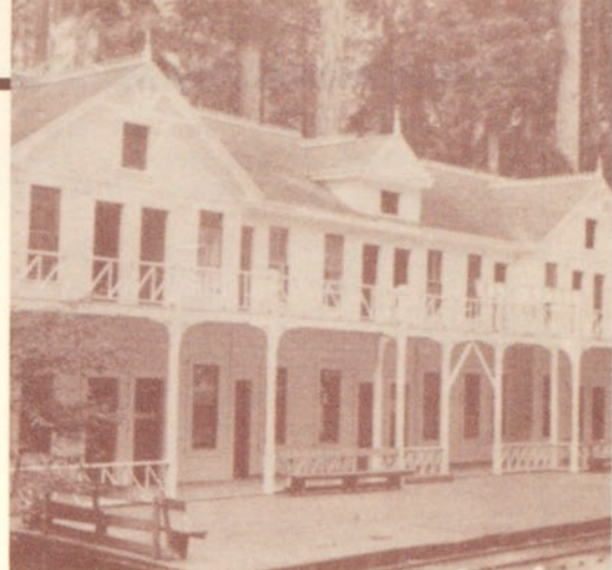
Passenger trains brought campers right to the front doors of Montgomery's Elim Grove Hotel at Cazadero, California.
