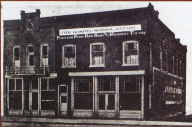
T. K. Leonard offered this storefront building in Findlay, Ohio, for the first headquarters of the General Council of the Assemblies of God.
