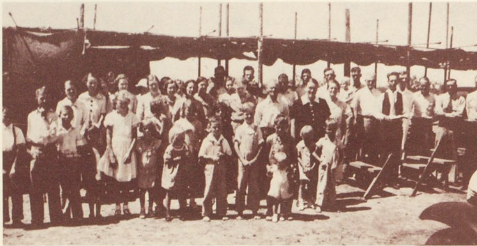
An unusual "brush" arbor which W. M. Panos and the author used at Brown Community, north of Big Spring, Texas, in 1936. With hardly any trees and brush around that part of Texas, they substituted 4-inch oil field boiler flues for the upright posts, pump rods (sucker rods) for the girders, and jute which was used to cover cotton bales for the roof.
